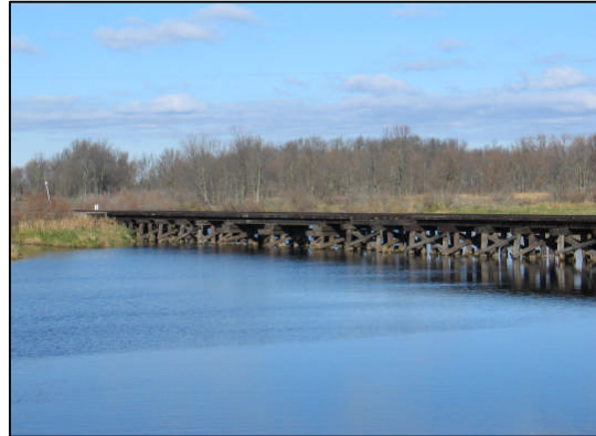
Railroad bridge, Village of Potter
